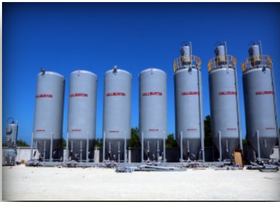
Dry Bulk Silos - Thailand
